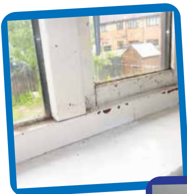
Steamy windows, black mould around window frames or on the backs of curtains?
